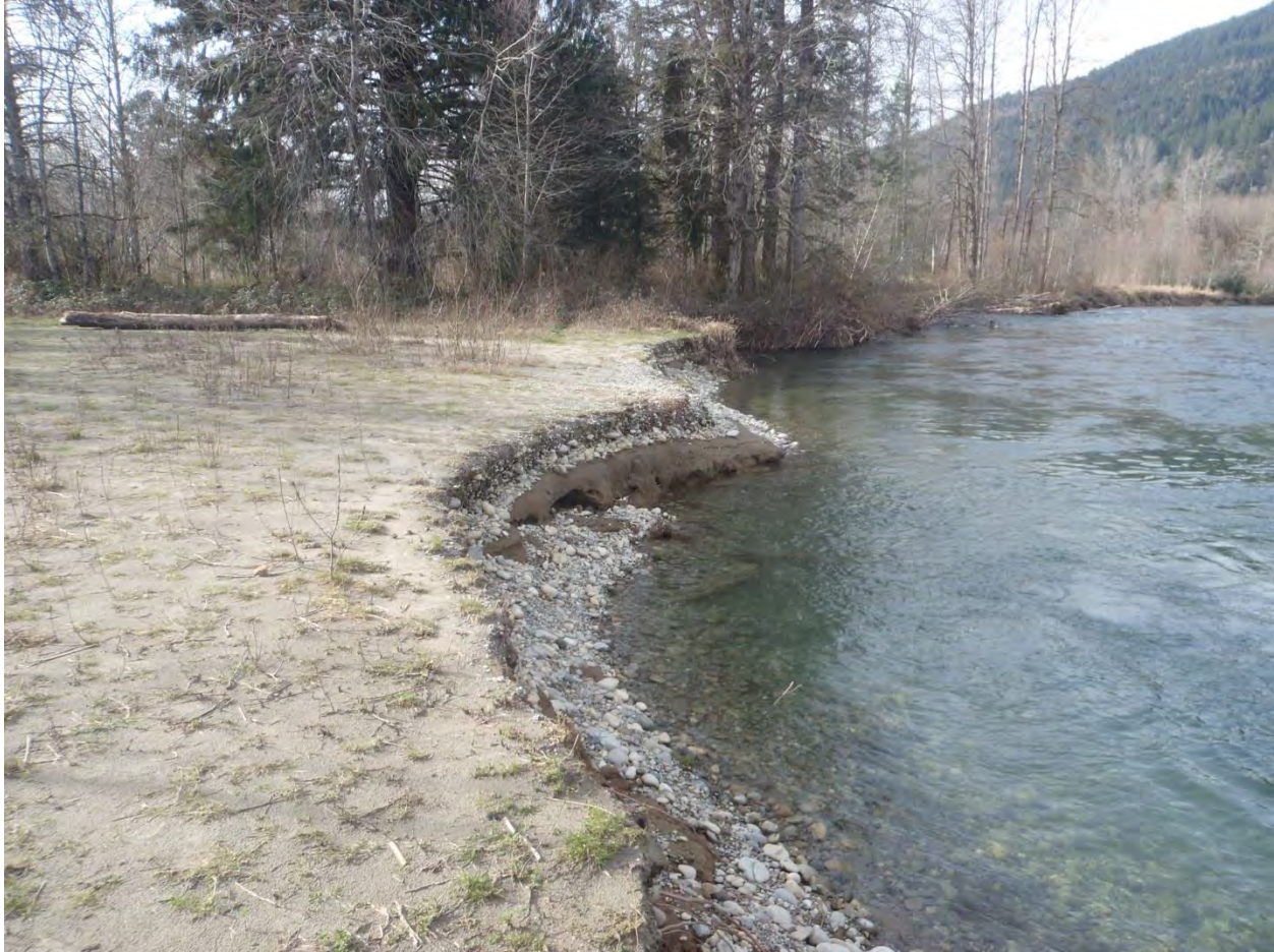
Figure 3 -Erosion Site at WDFW Access Point March 1, 2016
